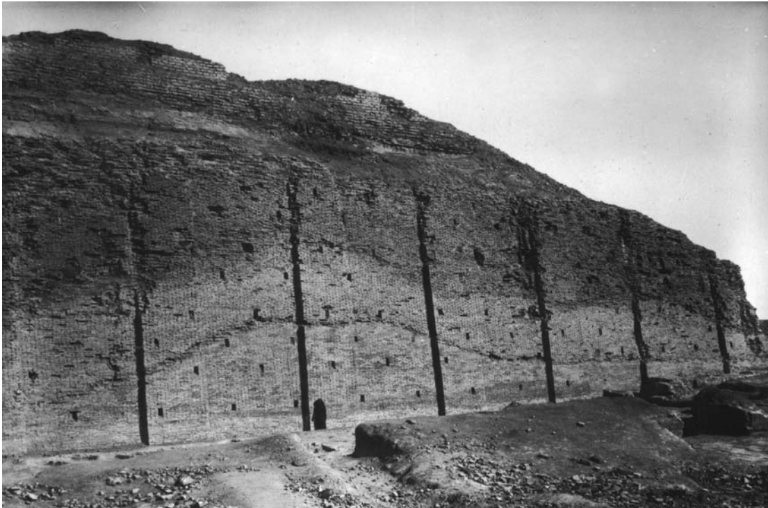
6.5 In this exterior view of the ziggurat at Ur, we can make out downspout channels and “weep holes” in the brick façade. These were designed to keep the interior of the structure dry. (University of Pennsylvania Museum)
